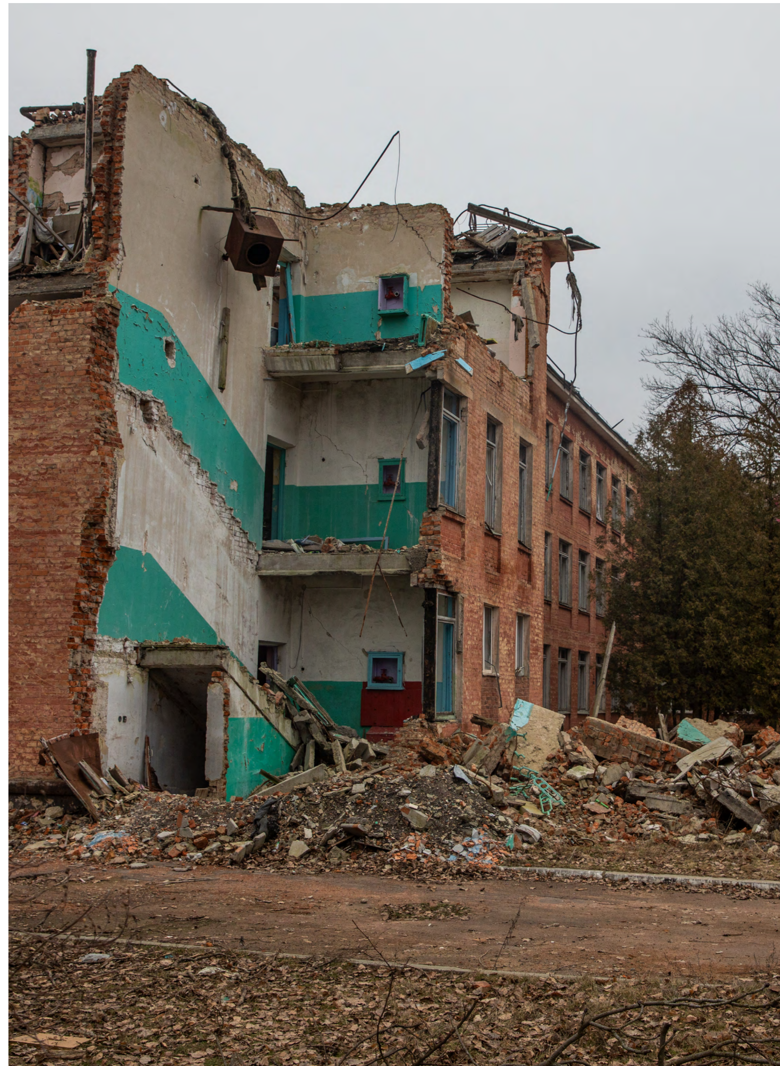
Ruins of a school in Chernihiv, Ukraine. This is one of two completely destroyed schools after missile attacks in the city. Photo taken on January 25, 2023 by Oleksandr Khomenko / Save the Children
