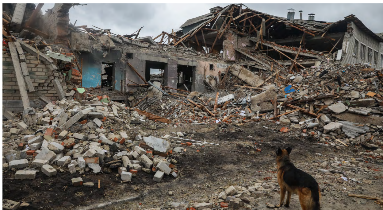
A school in a village near Kharkiv, Ukraine that was reduced to rubble by shelling. Photo taken on September 12, 2022 by Oleksandr Khomenko / Save the Children
